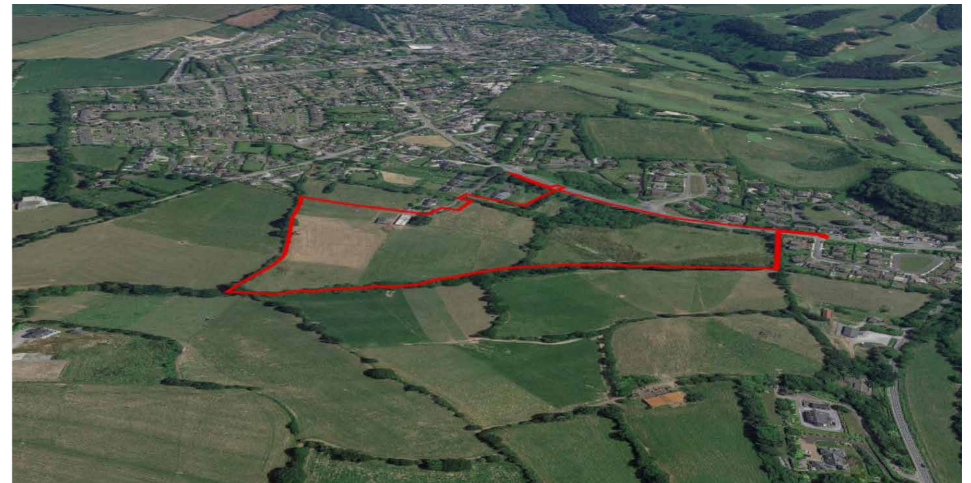
Aerial view from the west
