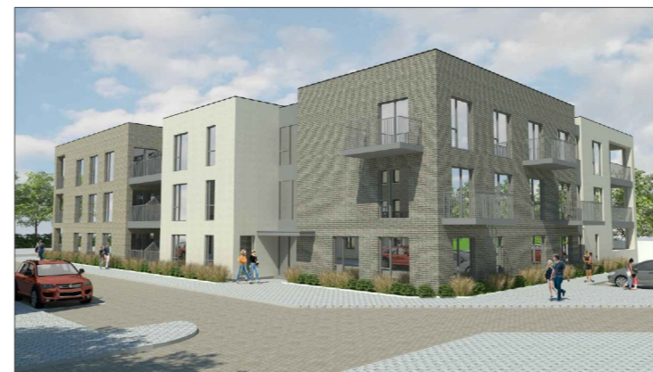
View of the north west corner
