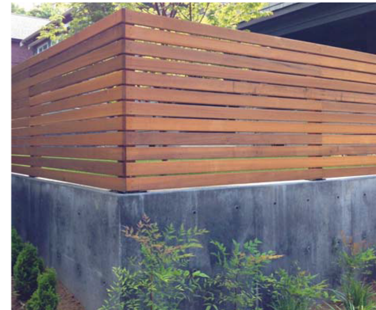
Example of conc. retaining wall topped with a timber panel fence. Proposed fence will be double-sided for presentation and full visual screening.
