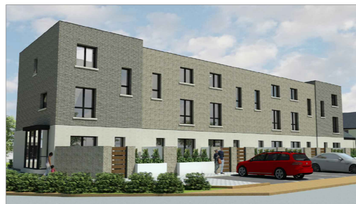
View of the eastern elevation
